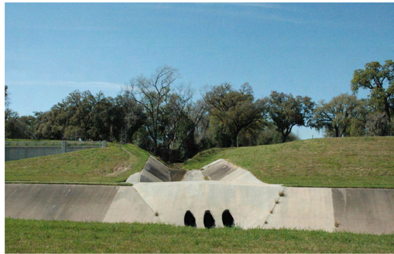
EXISTING CONNECTION FROM GOLF COURSE TO BRAYS BAYOU
