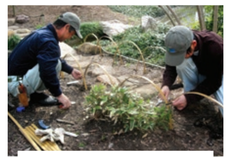
Hiroshi and Taiki Iwasaki construct a split bamboo fence along the stepping stone path leading to the tea house.
